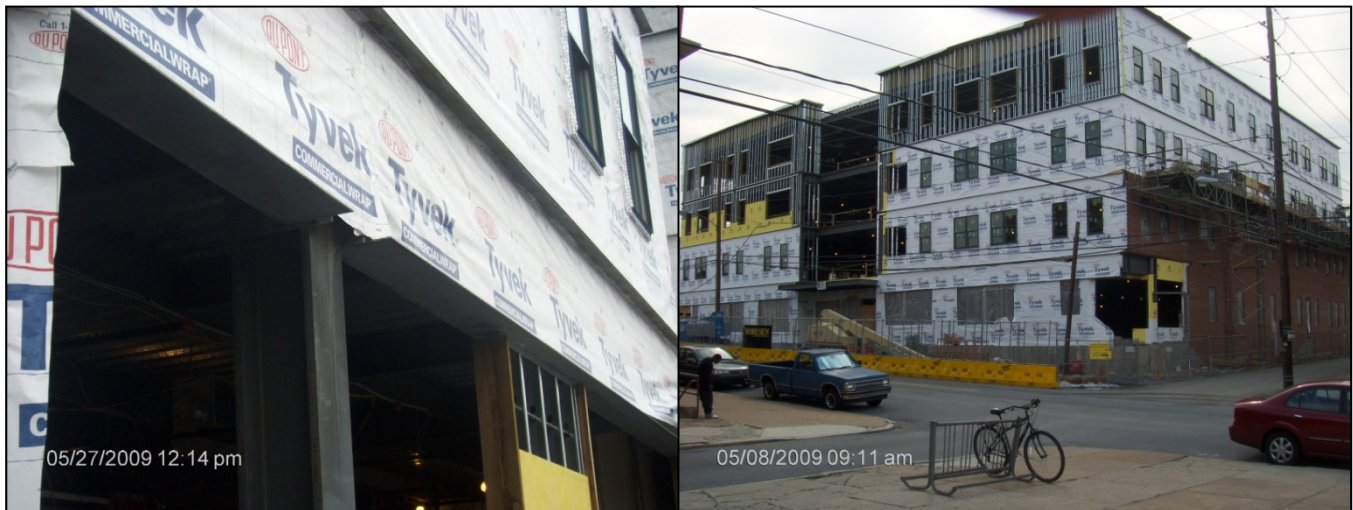
Figure 1 – Masonry Façade Steel Support Angles
